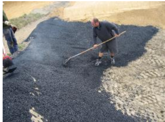
Hot asphalt being distributed with showels and by raking
