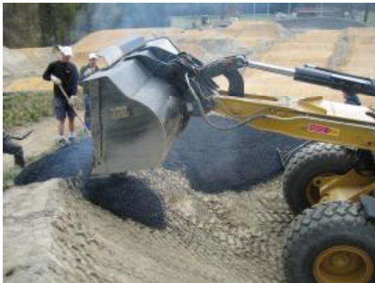
Asphalt is delivered
