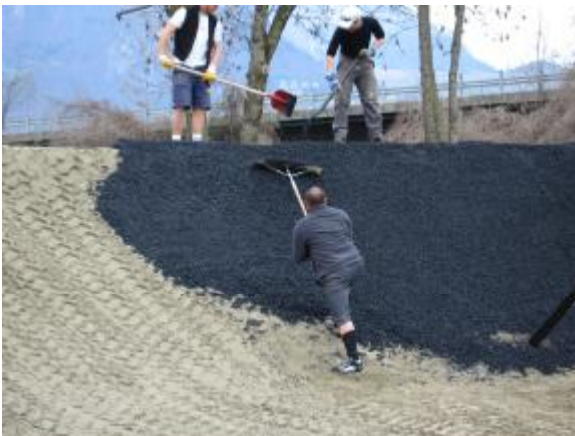
Asphalting turns is hard work
