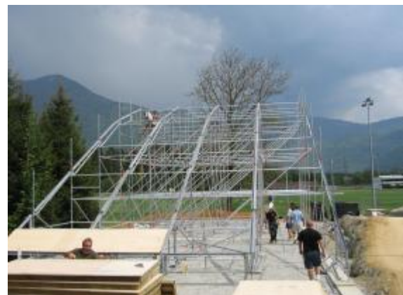
Start ramp assembly – Aigle, Switzerland
